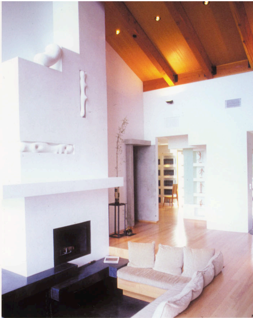
The roof of the living room and master bedroom (left) are constructed out of recycled timbers, detailed to create an exposed and honest expression of the framing and structural system and their connections.
