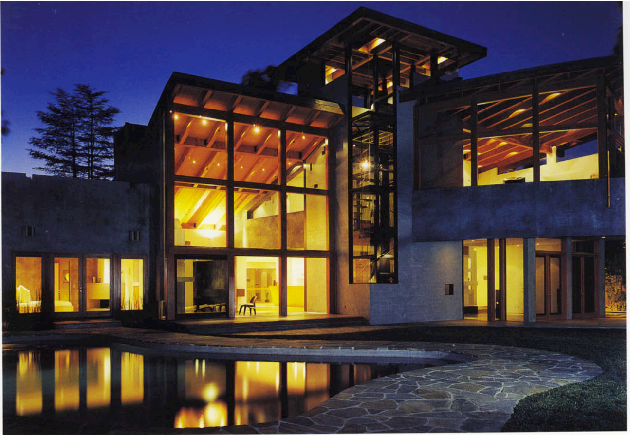
The 7,500 sq. ft. house is a case study in innovative environmental materials, methods and systems. Features include a solar domestic pool and radiant heating for slate floors, natural ventilation strategies, including heat recovery and exhaust by solar chimney, engineered wood products, trusses and steel framing, recycled lumber, high performance heat mirror glazing, cotton insulation and zero-VOC paint.
