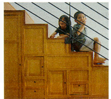
Sophie, 4, and Collin, 5, play on the Douglas fir stairs designed by Hertz to resemble a tansu chest and built by craftsman David Albert.
