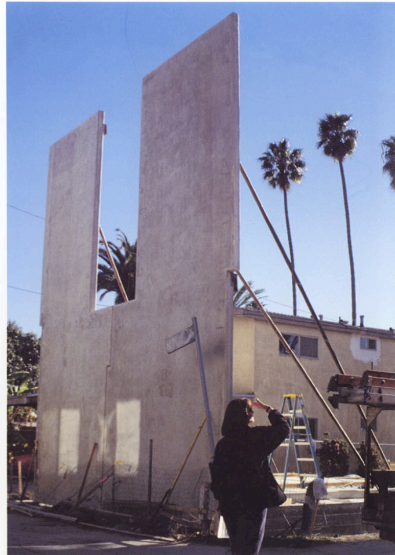
Hertz's design consisted of fourteen six-inch-thick tilt-up concrete panels facing each other along the longitudinal edges of the site, which composed an elongated interior space. The structure was erected in just ten hours.
